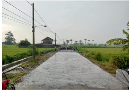
Figure 1. Construction of Corblok Dusun Donotirto RT 1 (Source: documentation of TPK Bangunjiwo)
