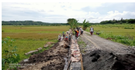
Figure 6. Talud construction reaches 80%
